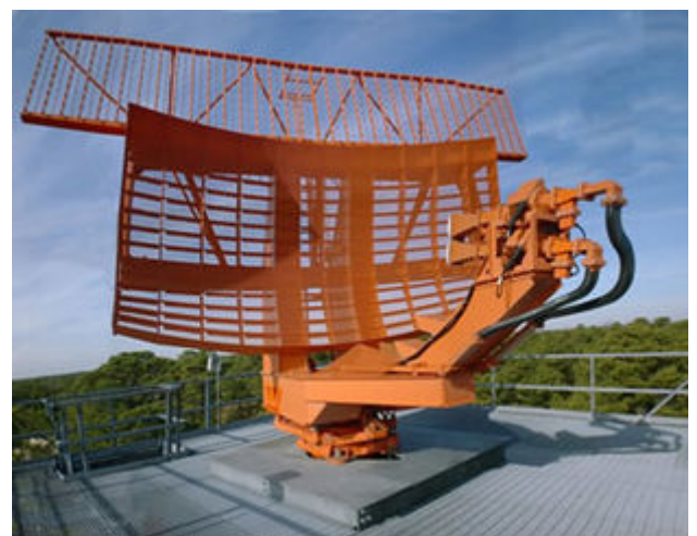
The parabolic antenna (lower curved surface) of an ASR-9 airport surveillance radar which radiates a narrow vertical fan-shaped beam of 2.7–2.9 GHz (band) microwaves to locate aircraft in the airspace surrounding an airport.
