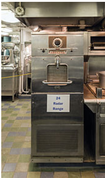
Raytheon RadaRange aboard the NS Savannah nuclear-powered cargo ship, installed circa 1961
