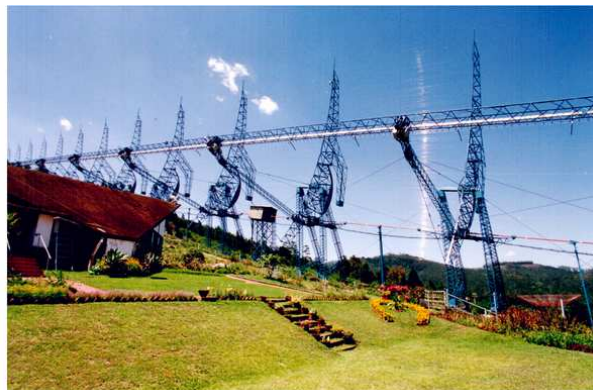
Fig. 5.3 ORT consists of a 530 m long and 30 m wide parabolic cylinder with its long axis parallel to that of the earth; the long white streak on right side is reflection of 1,100 stainless steel wires by the sunlight (Swarup et al. 1971)
