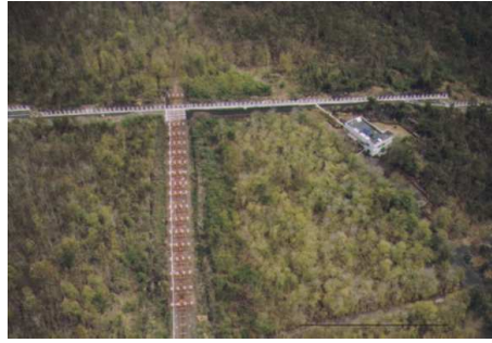
Fig. 5.27 An aerial view of the Mauritius Radio Telescope, as seen from the south. A part of the east-west arm with fixed helices is visible in the upper part of the figure. Sixteen trolleys with four helices each are seen in the south arm.
