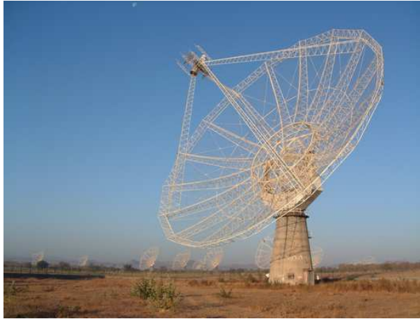
Fig. 5.5 A close view of a 45 m parabolic dish antenna of the GMRT. Ten far away antennas are seen in the background
