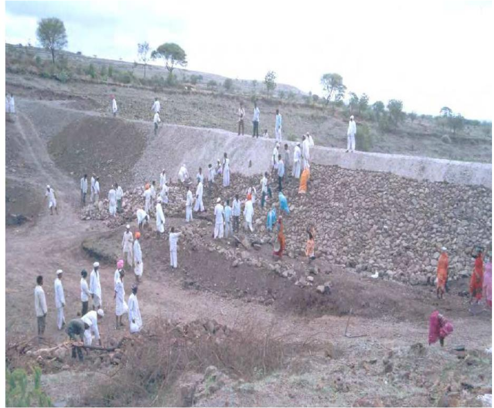
5. Stone pitching on the crest of the southern bank of a canal after the dam
