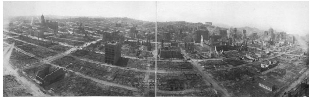
Aerial photograph of San Francisco earthquake damage - 5 May 1906 - collected from a kite
