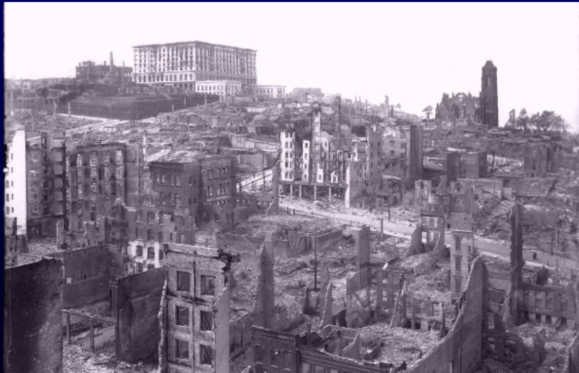
1906 San Francisco earthquake
