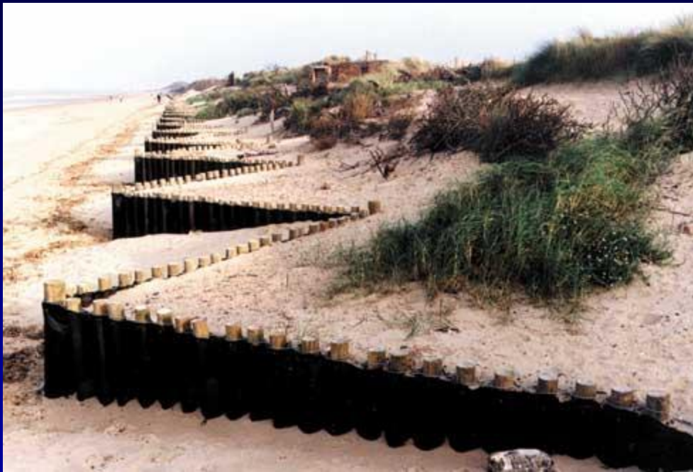
timber and geotextile
