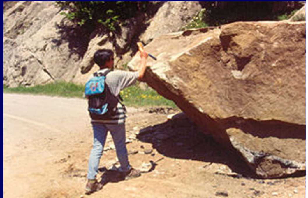
Castelmezzano - Italy. Landslide type: Rock fall
