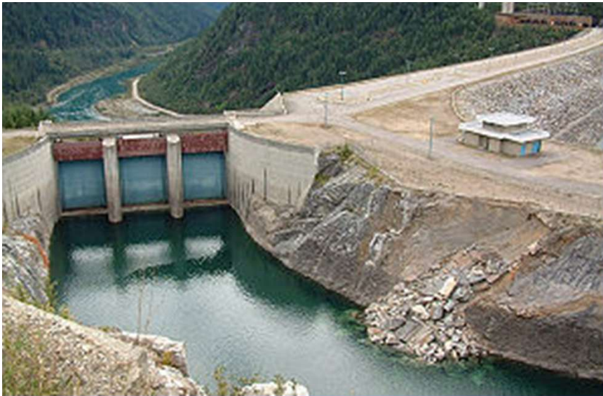
Canada Landslide type: Rock Slide
