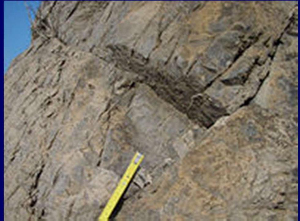
Lauria - Italy Landslide type: Wedge failure
