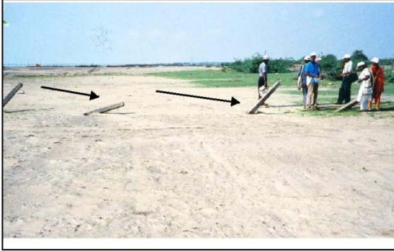
Deflected Pillars in Samiyapettai village (Nagapattinam area)
