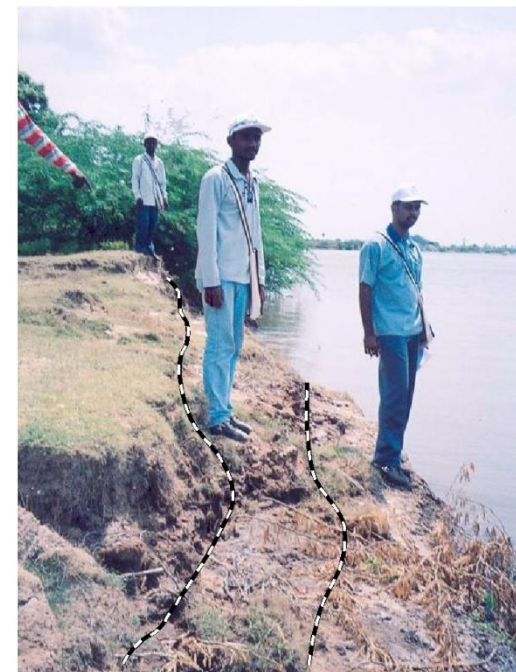
(A) Tsunami cut terraces in Uppanar river - Nagapattinam
