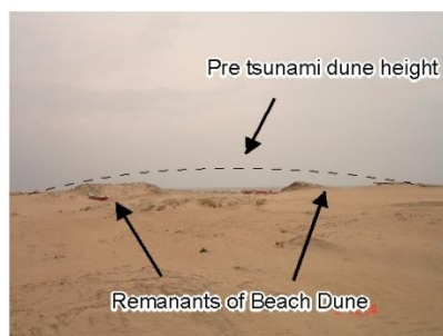
(D) Flattened beaches - Therkupoyyur village (Nagapattinam area)
