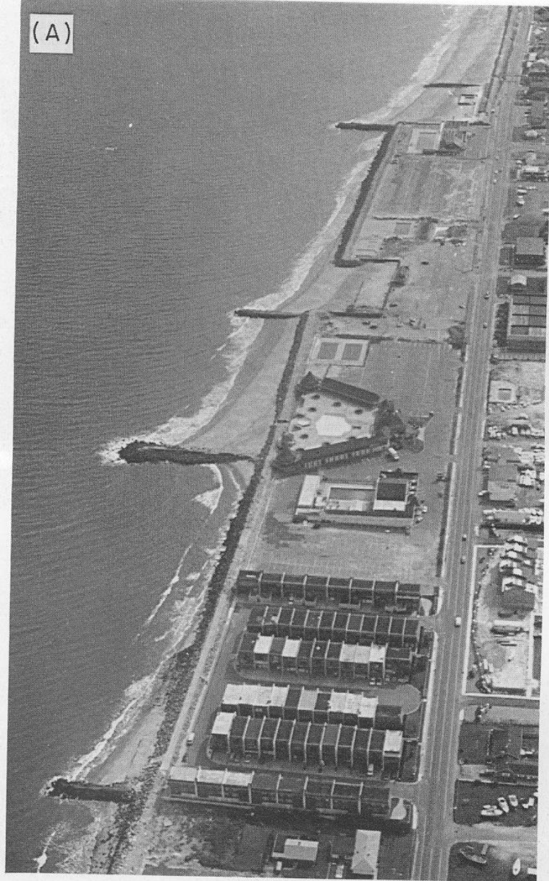
(A) Groynes on the sand-starved coast of northern New Jersey have little obvious effect on shoreline stability.
