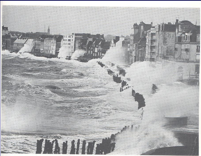
Figure 213. The vertical granite seawall at St. Malo in northern France during an onshore gale. Note the line of wooden posts aimed at reducing the direct wave forces on the wall, and the partial clapotis in the nearshore zone.
