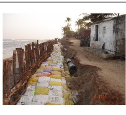
(B) Eroded beach being under protection - Pudupettai village (Nagapattinam area)
