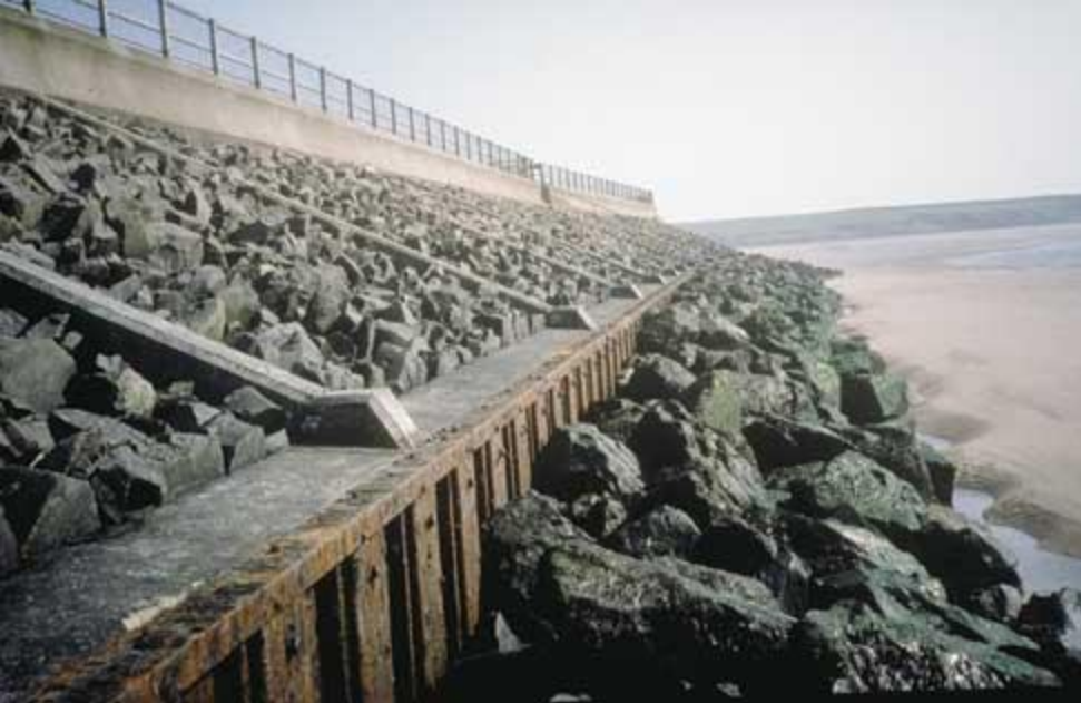
Rock faced concrete revetment
