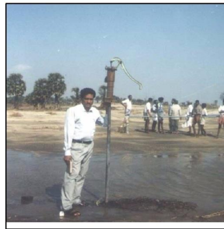
(C) Lifted handpumps - Cuddalore
