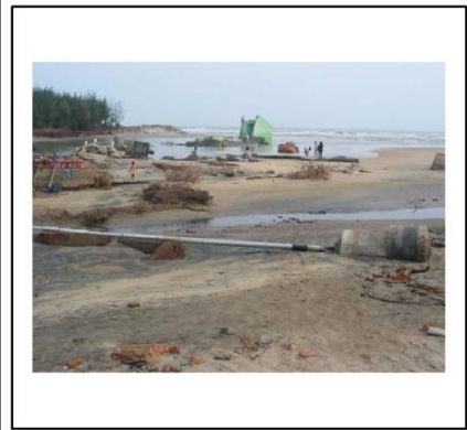
Collapsed childrens park - Nagapattinam
