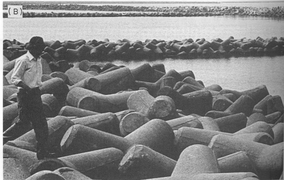
Figure 214. (A) Wire-frame gabions employed as a groyne system on a low-energy, macro-tidal coast in Norfolk, UK. (B) Tetrapods are used widely to protect the shore. Their large and irregular surface area helps wave dissipation, while the "legs" interlock to produce stability.
