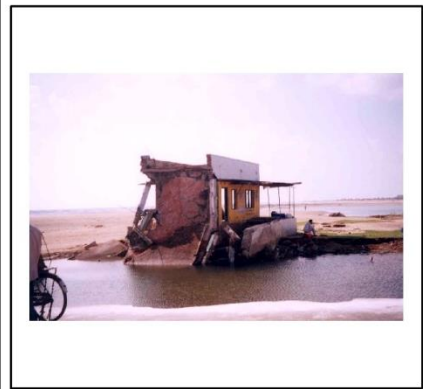
Damaged fish chilling plant - Devanampattinam (Cuddalore)
