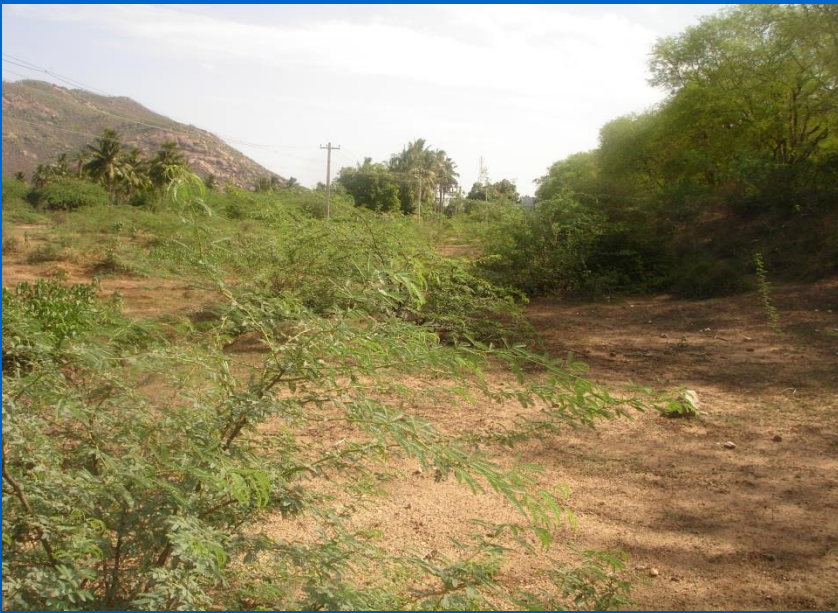
(1) TOTALLY DEFUNCT AND VEGETATED
