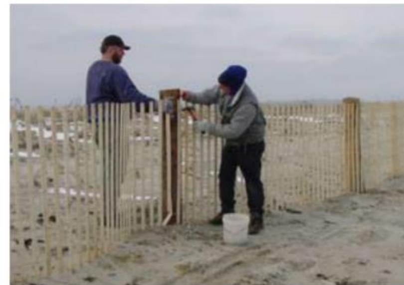
Figure 12. Fence is attached to 6" diameter posts.
