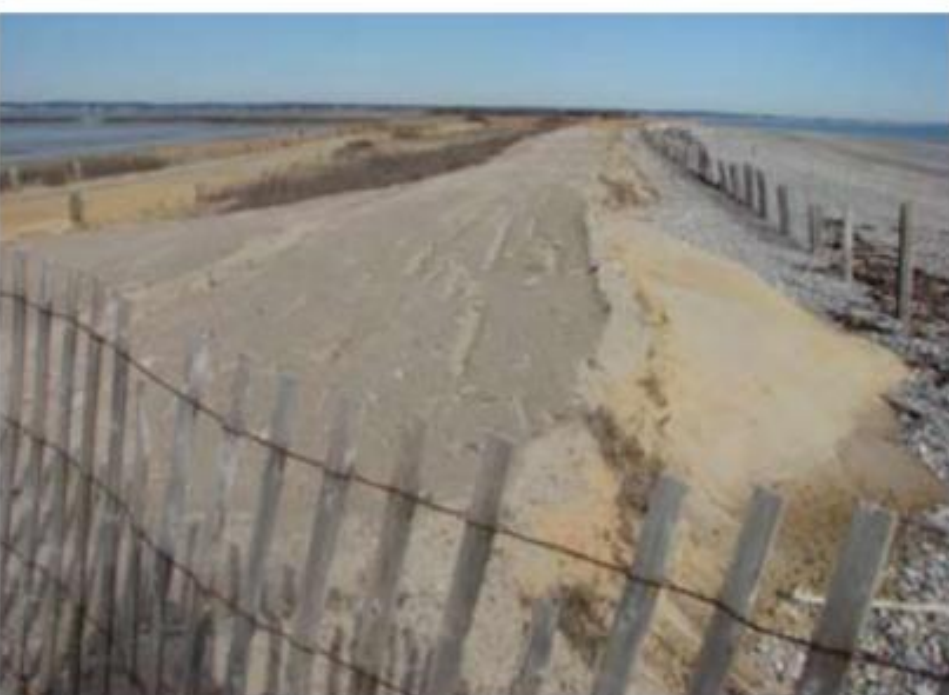
Figure 3. Covering quarry sand with natural dune sand.
